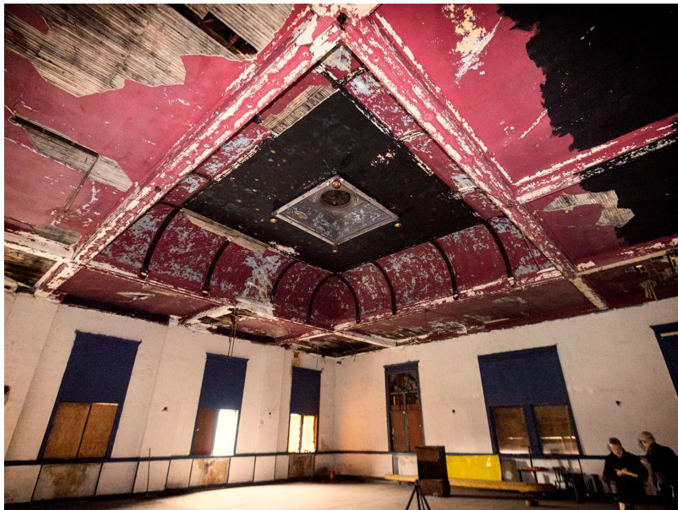
Inside Forum Hall on the second floor.
